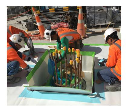
With three basement levels more than 17 metres deep, the Commercial Bay project required a waterproofing solution that would work in a wet and muddy environment while addressing the complex architectural design. At the same time, the solution had to form a permanent, continuous seal against water and a barrier to resist the stress of ground settlement.
