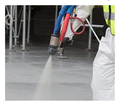
Prior to reconstruction, Tab Associates needed to find a weather barrier that would do the job. They needed the barrier to be seamless, to seal around fasteners, and be impermeable to liquid water. In addition, since the previous moisture barrier had been incorrectly installed by the original architect, Tab Associates wanted to find a product supported by technical services that would help them do the job right the first time.
