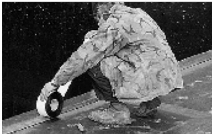
Joints between boards primed and Armour tape applied
